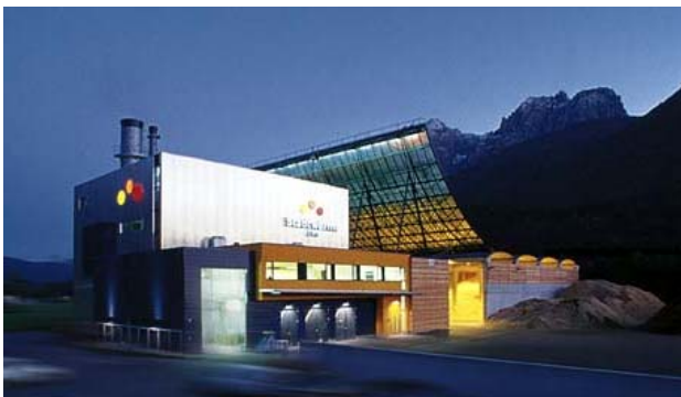
Figure 3: Comparably sized biomass CHP plant with fuel storage, administrative offices, and solar thermal preheat
