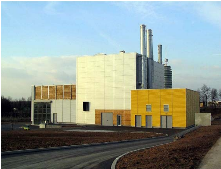
Figure 5: Comparably sized biomass CHP plant with fuel storage, and administrative offices
